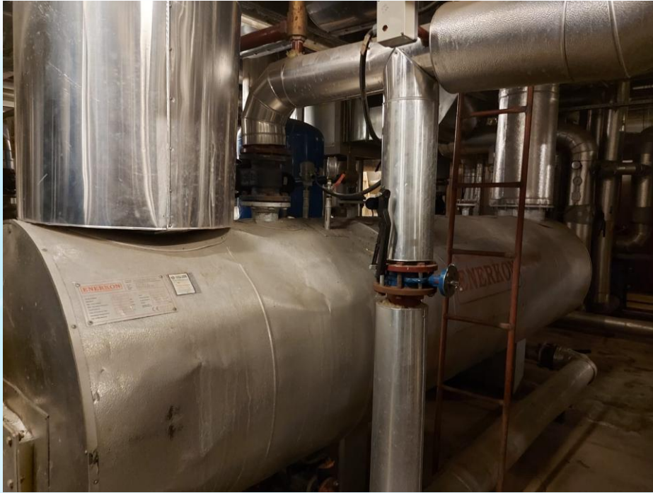
Figure 3. Exhaust gas-hot water heat exchanger
