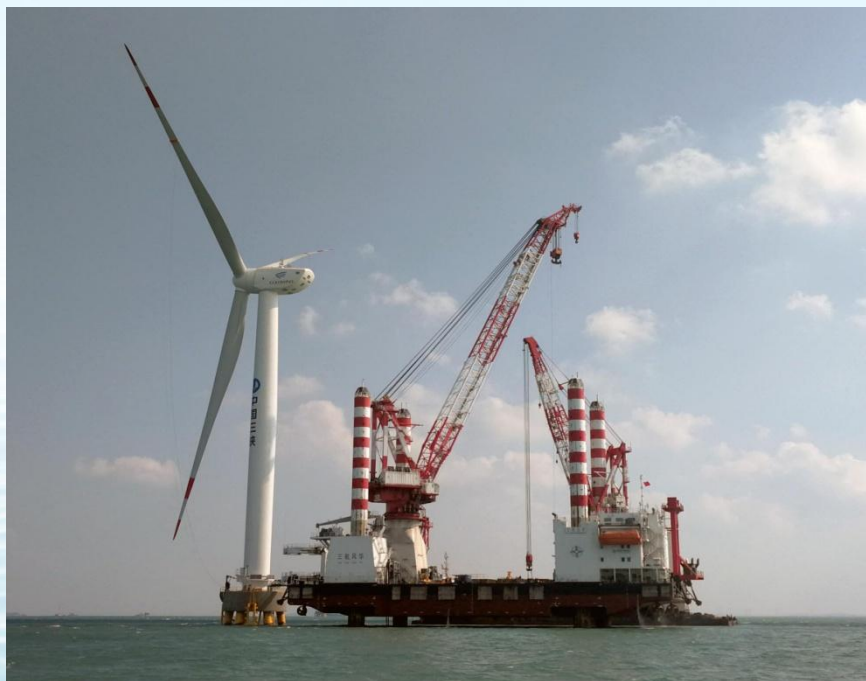
Figure 1. The 1000 ton jack up wind turbine installation ship.
